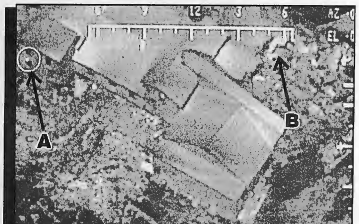
Still photo at 12:04:55 p.m. Central Standard Time from FBI's FLIR video shows: (a) heat plume on second floor at southeast corner of complex — FBI cites this as first point of ignition in fatal fire; (b) heat plumes spreading out through rubble of collapsed gym, possibly indicating early point of ignition.
